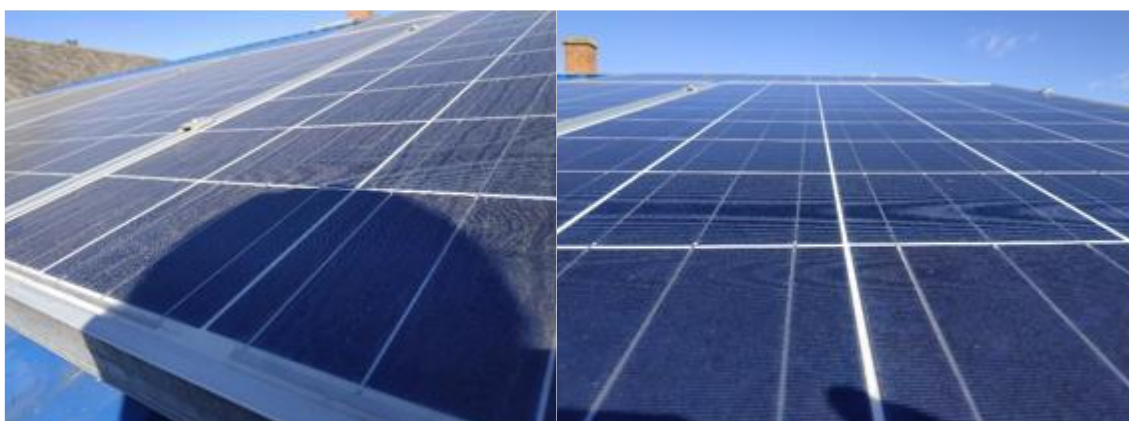
6 Figure: The ninth day was dirty solar panel (left) and post-rain solar panel (right).
